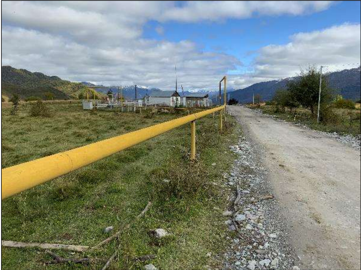
Figure 45: Didveli Plateau, approximately KM 1
