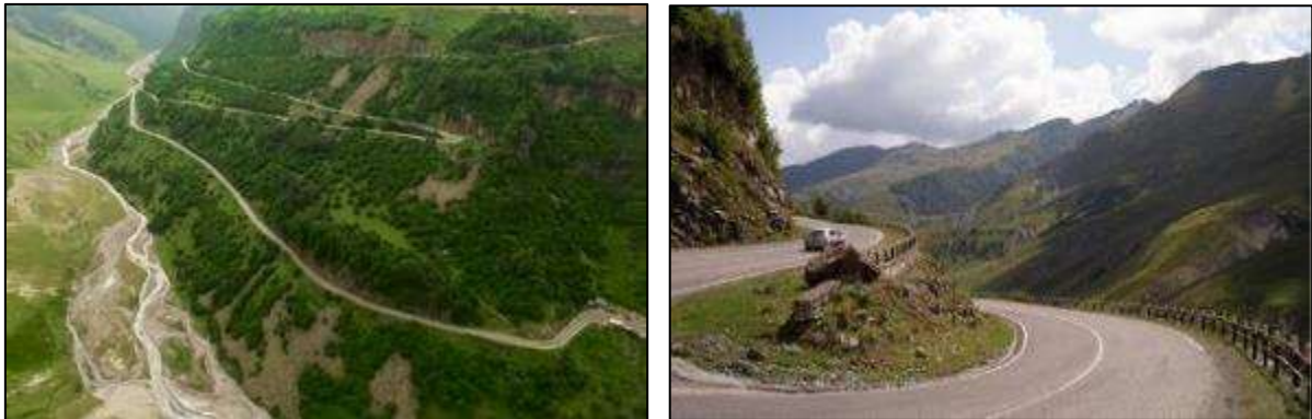
Figure 13. Existing Road Conditions
